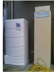
Plug and play solar cylinder+gas
